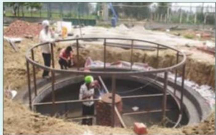
Fixing of guide frame for placing M. S. Gas holder
