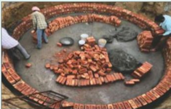
Construction of pit for placing M. S. Gas holder
