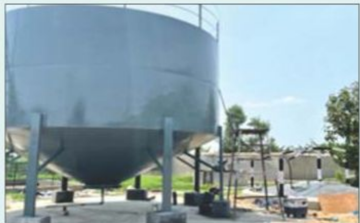
Overall view of biogas plant
